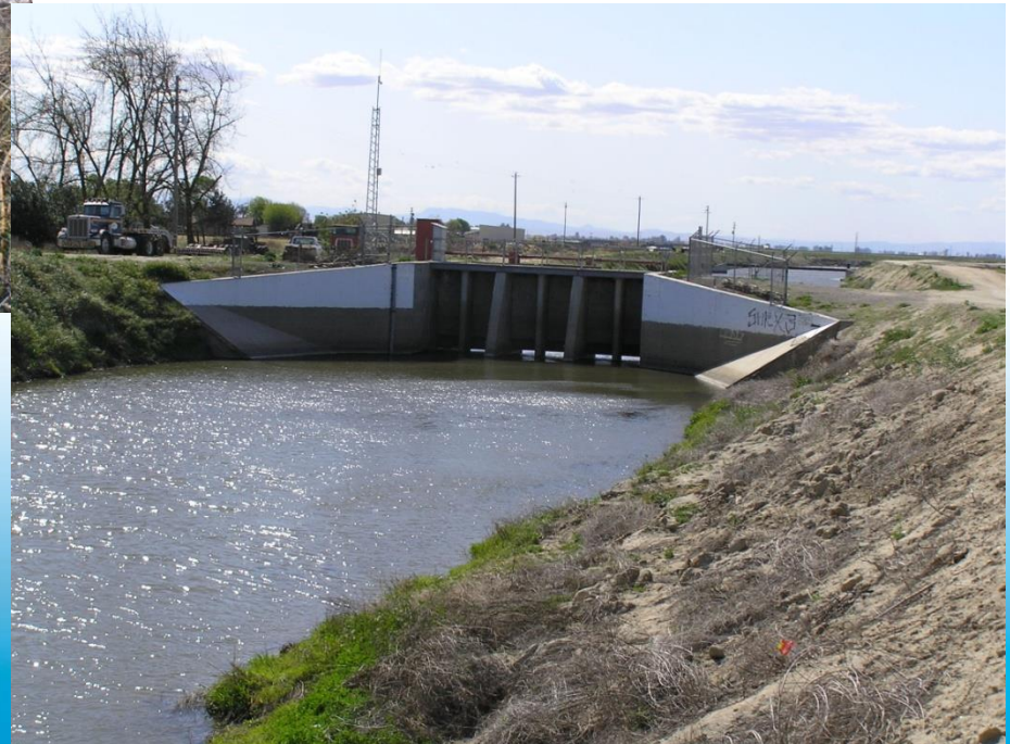
Arroyo Canal – Screen to prevent fish entrainment
