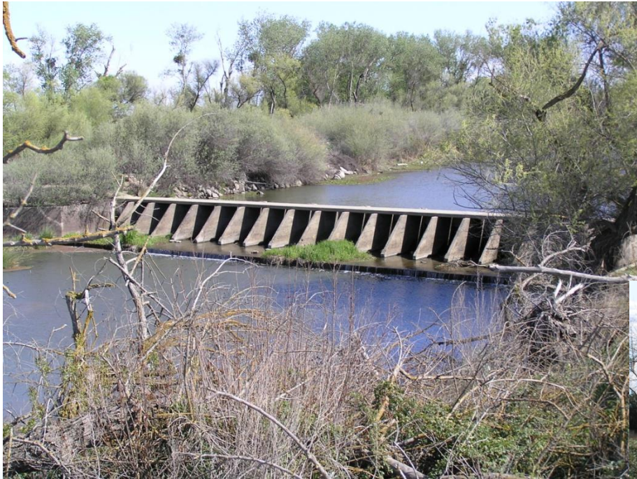
Sack Dam – Modify for fish passage
