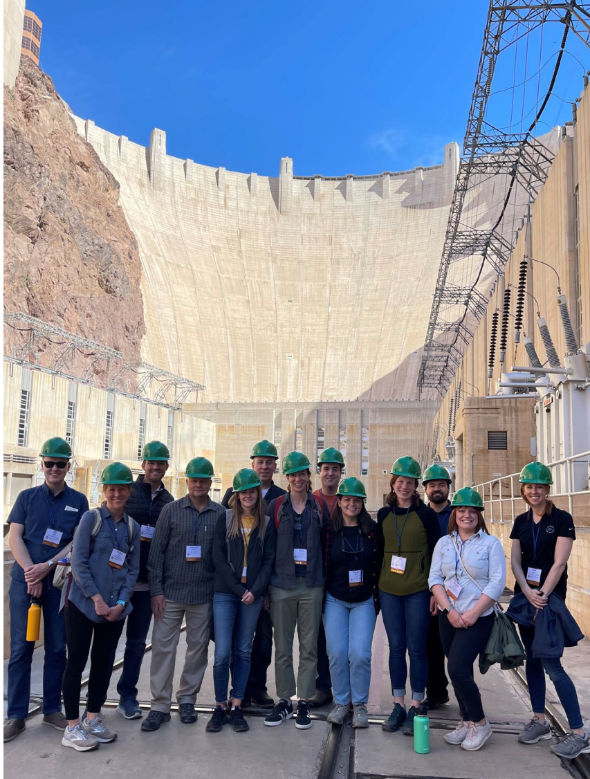
Colorado River Water Leaders at Hoover Dam, a stop on the Water Education Foundation's Lower Colorado River Tour in March 2022.
