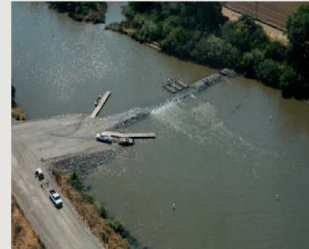
Temporary Barrier: Grant Line Canal
