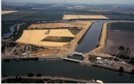
Permanent Barrier: Delta Cross Channel Gates (photo courtesy of USBR)
