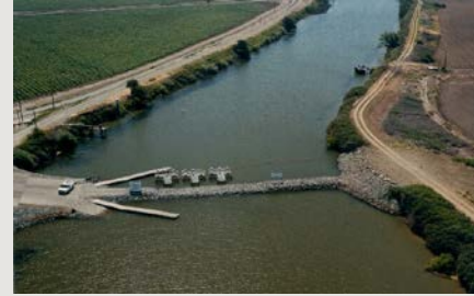
Temporary Barrier: Old River at Tracy Blvd.
